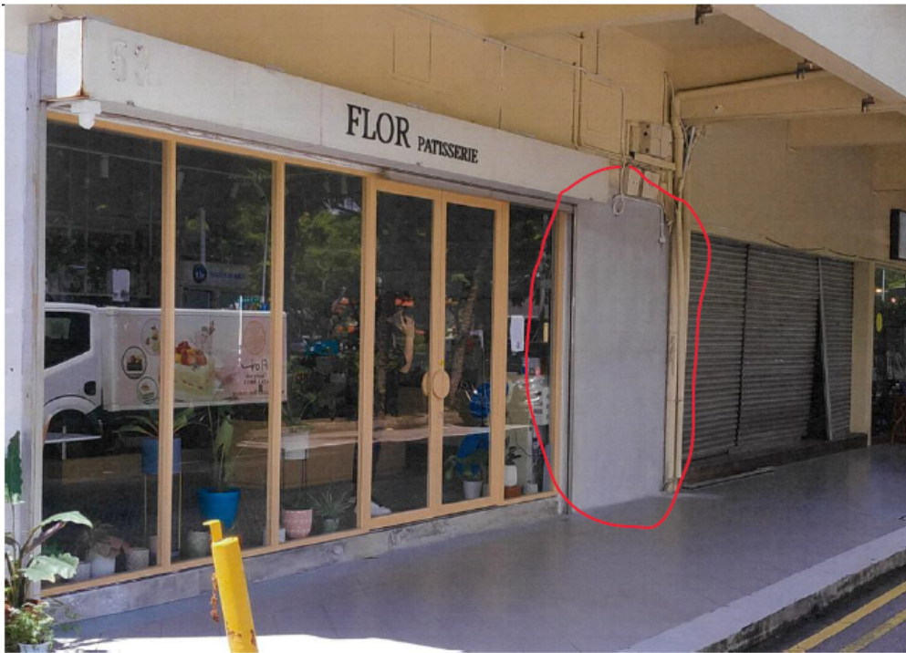
Figure 4: Side view of the front wall of Unit 53
