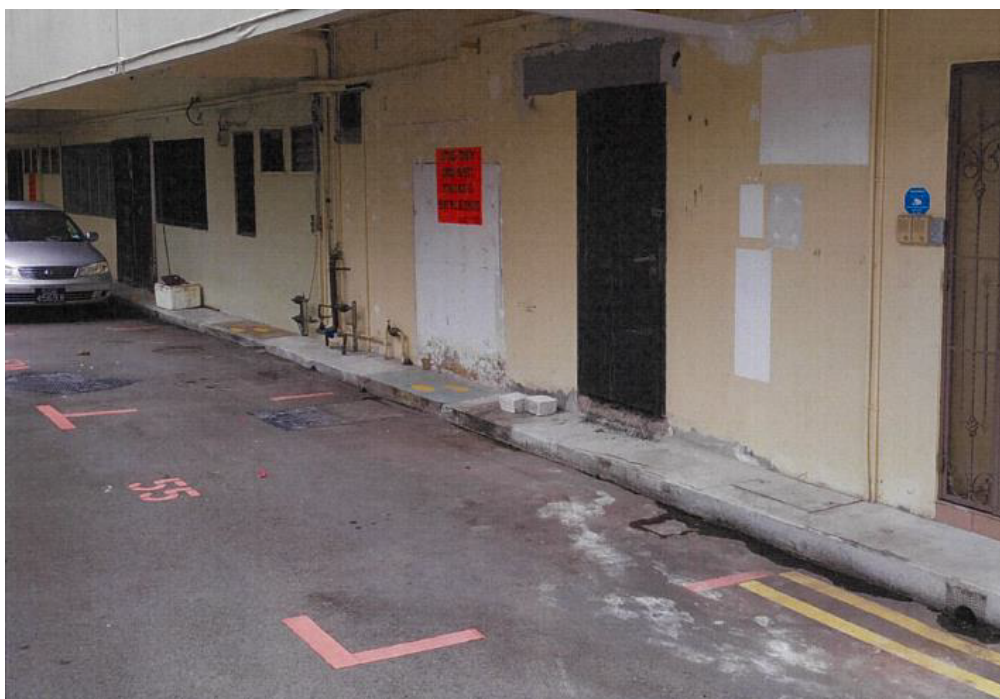
Figure 1: Current state of the rear of Unit 53
