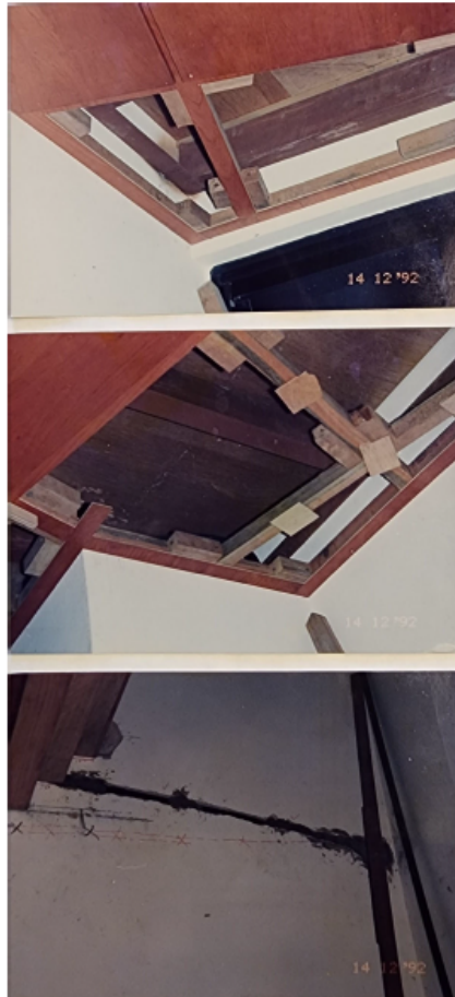
Fig. 5: Photographs allegedly showing the installation of the mezzanine attics dated 14 December 1992
